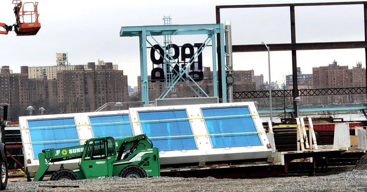
Figure 8. A truck full on concrete panels with windows inserted, ready for attaching to the building
