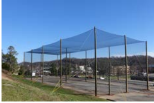
Outdoor Netted Enclosure
